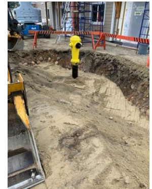
7 th Ave., Low-income hydrant installation
