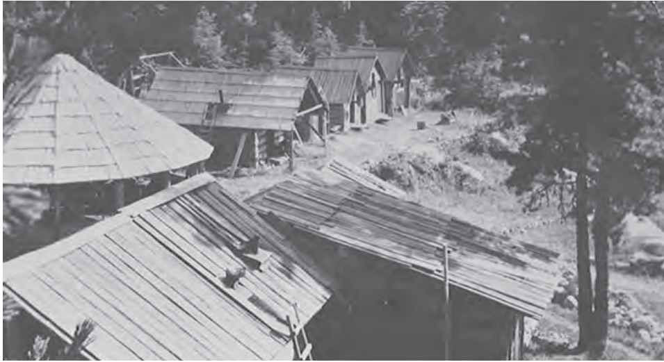
The original hot springs cabins at the source Photo: Nakusp Hot Springs
