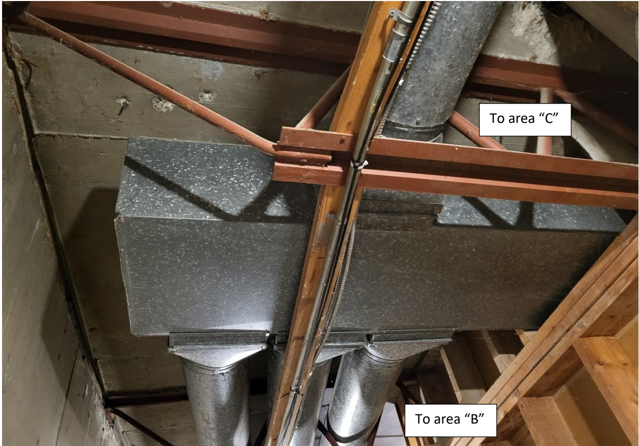
Image 14: Coming from mechanical room and splitting into area "C" and area "B"
