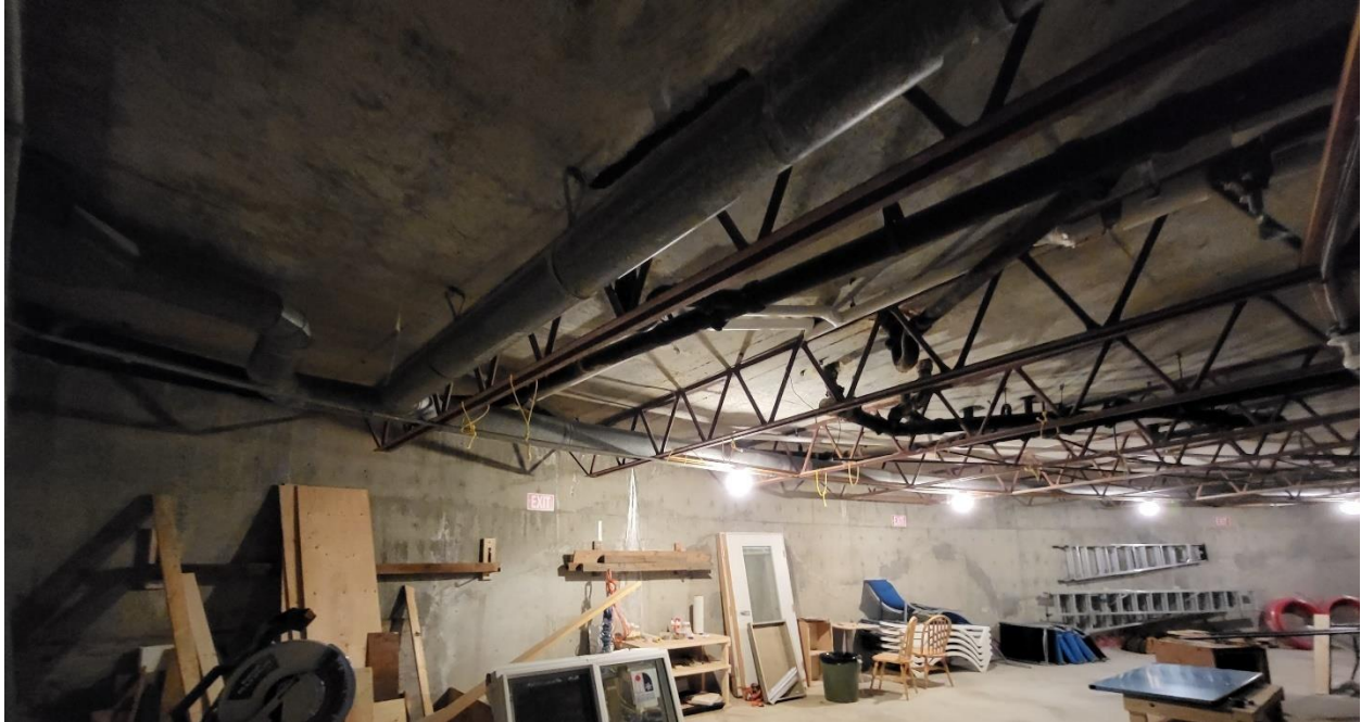
Image 13: Ductwork in area "C"
