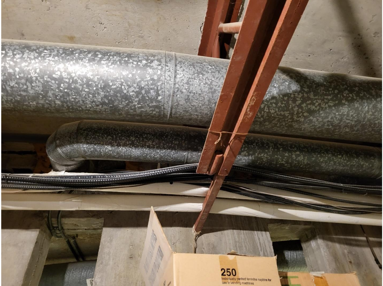
Image 21: Ductwork in area "A"
