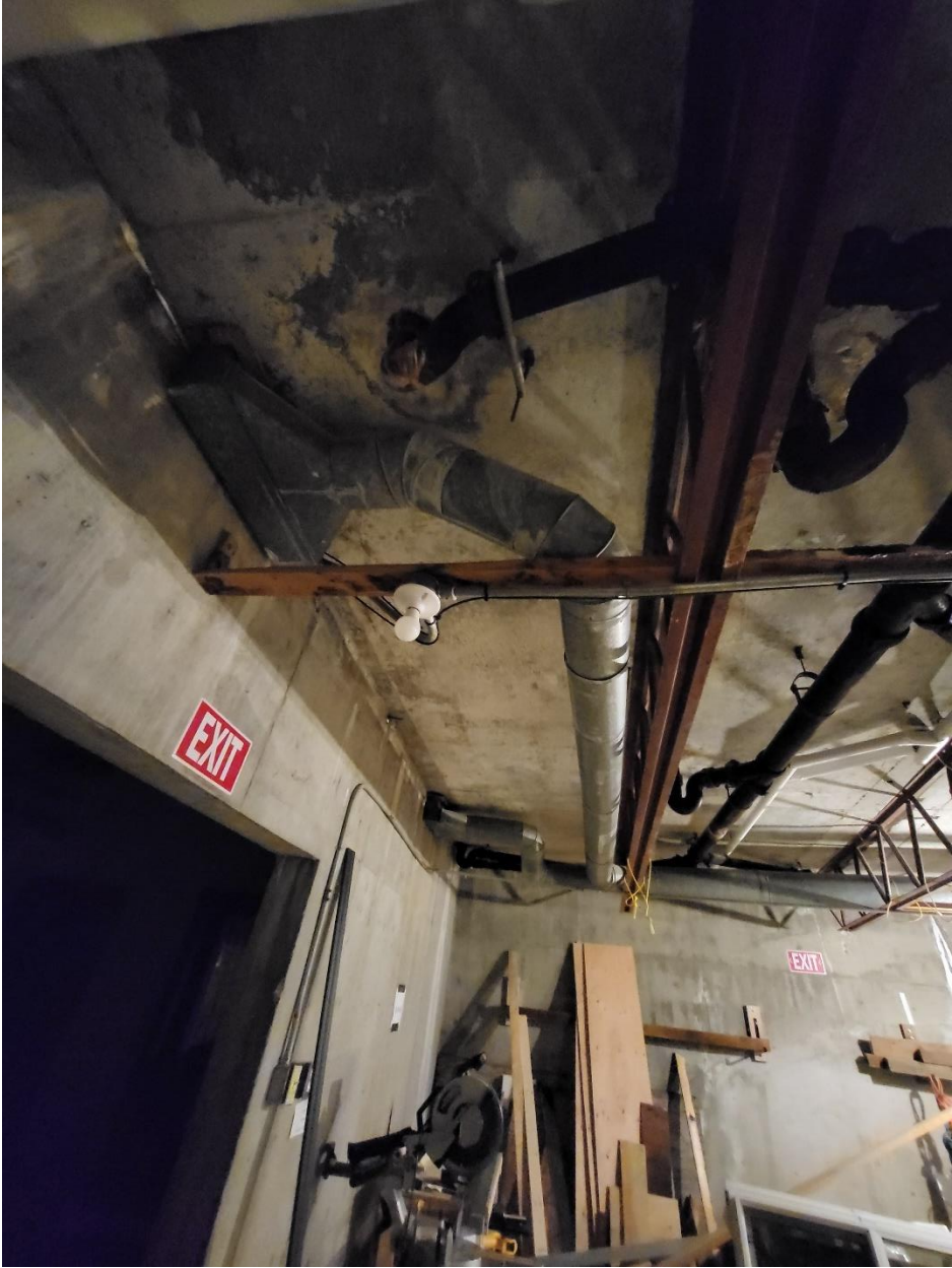
Image 12: Ductwork in area "C"
