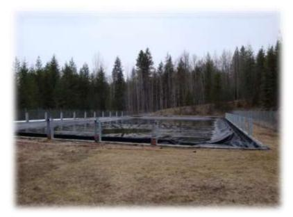
Chlorine is combined with surface water and then stored in the million gallon reservoir. The reservoir has a polyvinyl chloride cover to keep out debris and wildlife. Towers and weights around the perimeter allow the cover to move with the water level, The reservoir is 14' deep.
