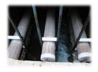
clogged, especially during the freshet and require monitoring and cleaning. Course filtration is not technically considered a treatment process, as fine materials and micro-organisms are not removed, therefore, chlorination is required.
